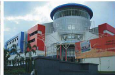
Indonesia Plaza Asa project, Tasikmalaya
