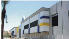
Saudi Arabia Al Qasr Project
