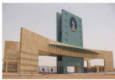
Saudi Arabia Hall University Project
