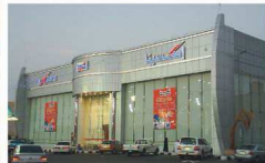
Saudi Arabia Elasa Center, Jeddah
