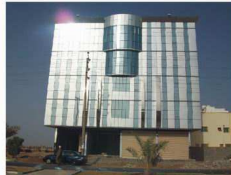
Saudi Arabia Commercial & Residential Building, Raigh
